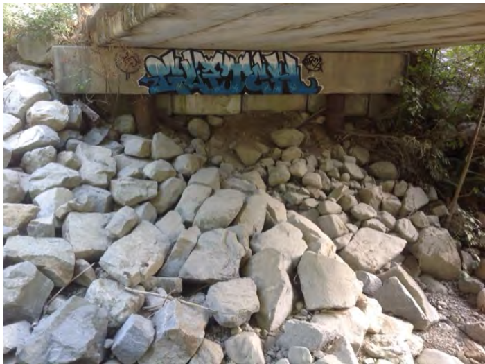
Left Bank Abutment when facing downstream
