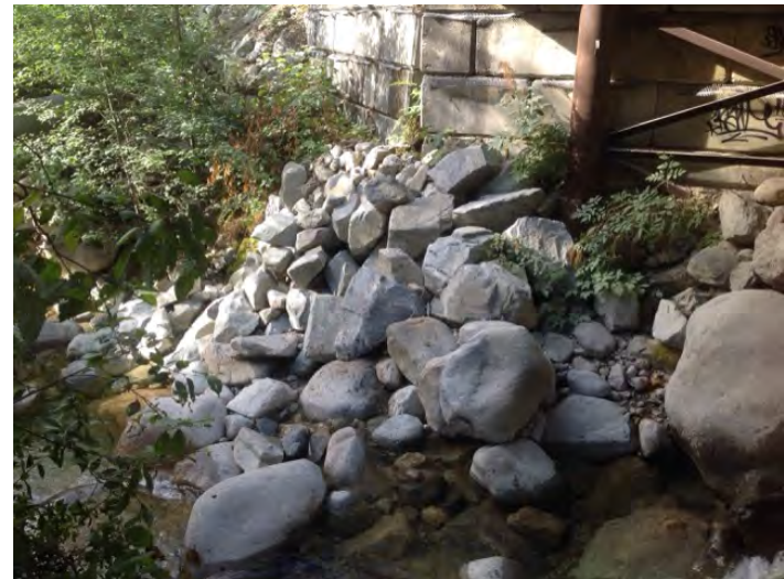
right downstream abutment
