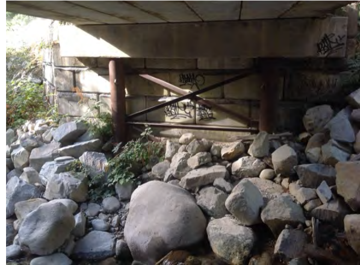
Right Bank Abutment when facing downstream
